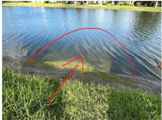
8136 – 8131 Victoria. Unburied downspouts above washout trench & silt build up in pond
