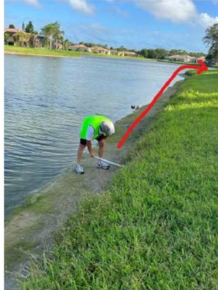
9 – 13" undercut cavity from 8139 through to E/W arm to 8055 Victoria
