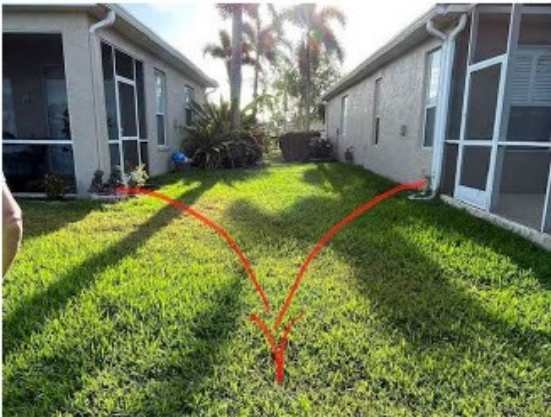
8136 – 8131 Victoria. Unburied downspouts above washout trench & silt build up in pond
