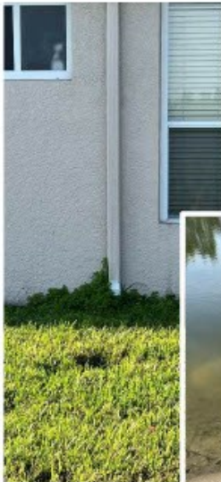
4281 buried drainpipe/continued erosion/silt around pipe opening.
