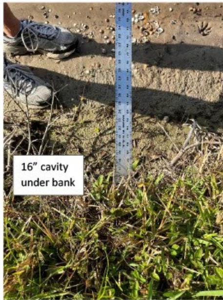
North side of Pond 8 across from 8154 Victoria. 16" deep cavity under the bank with signs of bank collapse below planted bed. Evidence of animal burrows that can increase soil instability and erosion.
