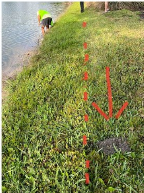
North side of Pond 8 across from 8154 Victoria. 16" deep cavity under the bank with signs of bank collapse below planted bed. Evidence of animal burrows that can increase soil instability and erosion.
