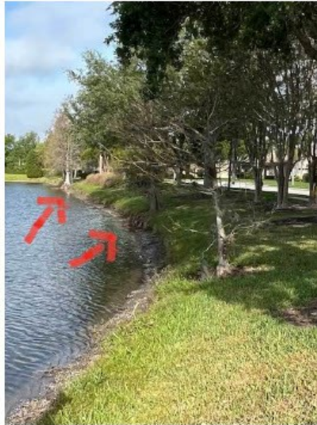
North side of Pond 8 across from 8154 Victoria. 16" deep cavity under the bank with signs of bank collapse below planted bed. Evidence of animal burrows that can increase soil instability and erosion.
