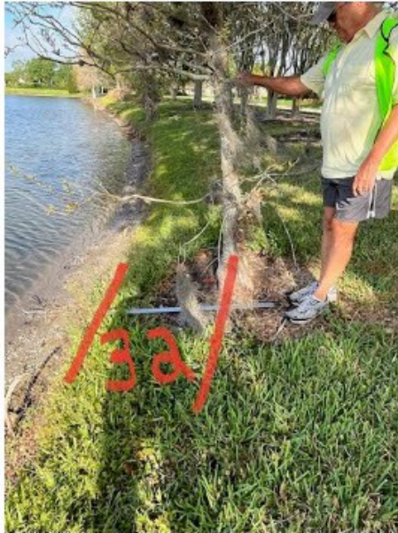
North side of Pond 8 across from 8154 Victoria. 16" deep cavity under the bank with signs of bank collapse below planted bed. Evidence of animal burrows that can increase soil instability and erosion.
